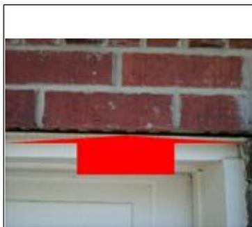
Separation at the lintel and the brick above garage door.
