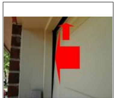
Garage door has large gap on left side. Should be flush.
